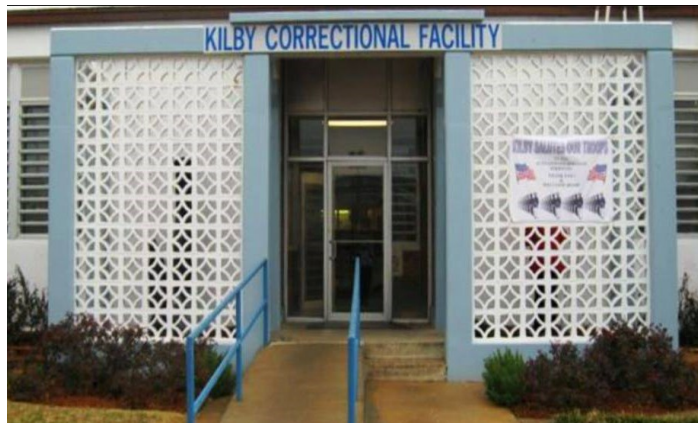
The Kilby Correctional Facility —1969 Renamed in honor of Thomas E. Kilby who was Governor when the first Kilby Prison was constructed in 1923. Kilby is the male intake and reception center.
