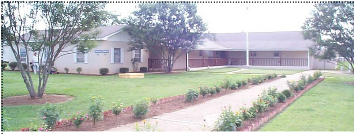
Red Eagle opened in 1972 and is currently a community work center.
