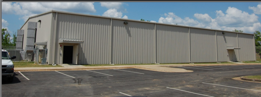
New ACI Sewing Plant at Wetumpka Women’s Facility
