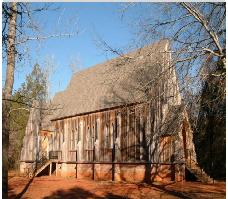
St. Luke's Episcopal Church (circa 1854) relocated and restored at Old Cahawba by ACI Construction & Remodeling crews.
