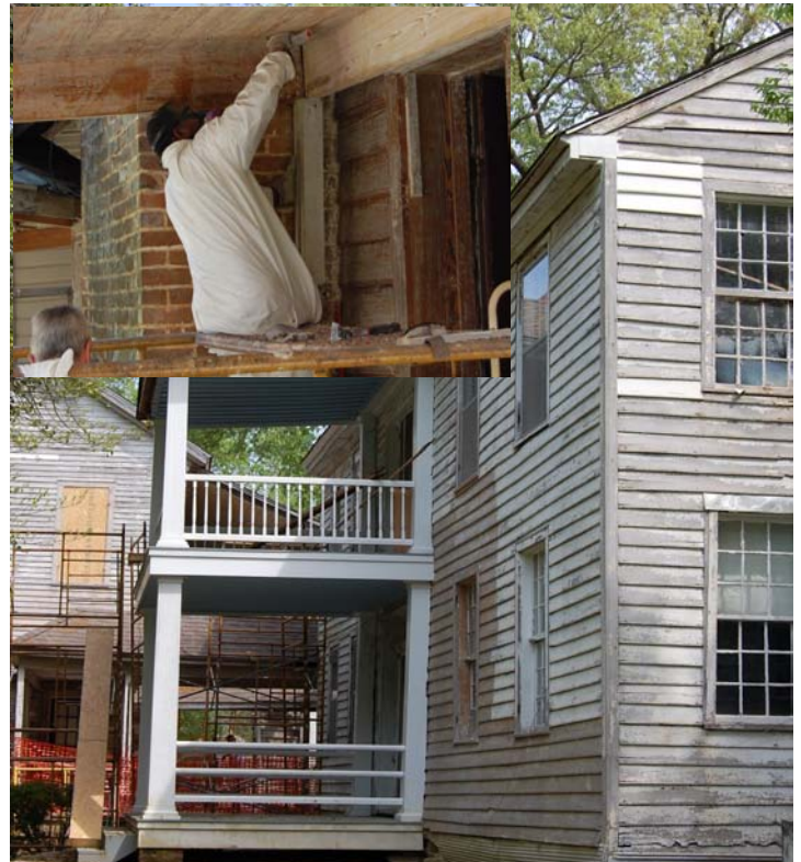
Architectural restoration and lead-based paint abatement being conducted by ACI crews at Joe Wheeler house near Courtland for the Alabama Historical Commission.
